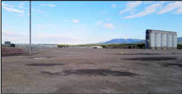
Pictured above are former potline buildings with remaining ore silos visible.
